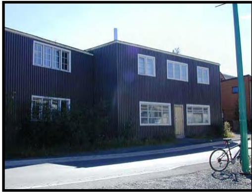
Hudson's Bay Warehouse.
